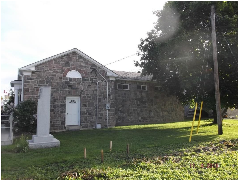
South Side of the Building showing Extension to be added
