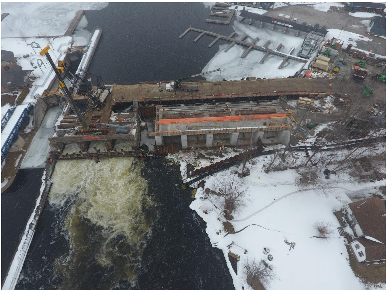
Port Severn Main Dam – March 6, 2020
